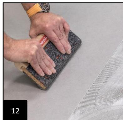
In order to achieve an optimum installation result, the covering must be carefully rubbed from the centre to the sides immediately after it has been placed (11) in the adhesive bed. (e.g. cork or surface scraper) from the centre to the sides (12).
