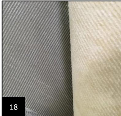
Afterwards, but not later than 30 minutes after manual rubbing, the covering is evenly and slowly rolled (17) using an articulated roller (weight min. 50 kg / 110lbs). Check that the covering is sufficiently wetted (18) with adhesive.
