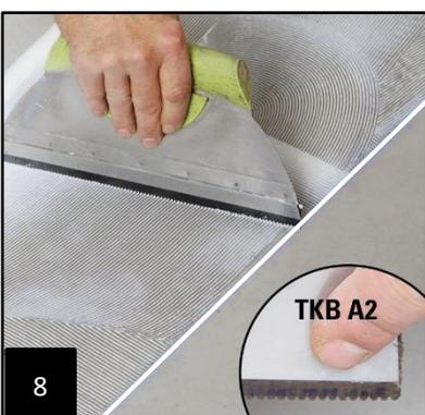
Now apply the adhesive approved by Windmüller GmbH evenly and lane by lane according to the adhesive manufacturer's instructions using the TKB toothed strip (usually TKB A2 toothing) recommended for this purpose (8).
