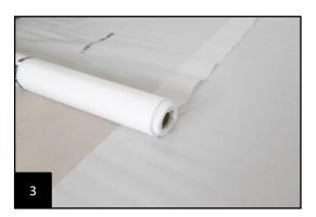
Subsequently, use the footfall and walking sound reducing insulating underlays recommended by Windmöller. For floor coverings with a laminated insulating carpet pad, also proceed as described above. Insulation underlays reduce sound transmission to other rooms, reduce footfall noise and thus significantly improve living comfort. The CS value (compressive strength) of insulation underlays should be at least  $\geq$  90 kPA.
